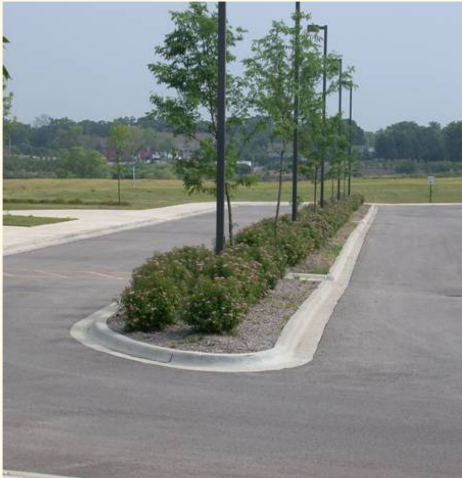
Typical parking lot island raised above pavement.
