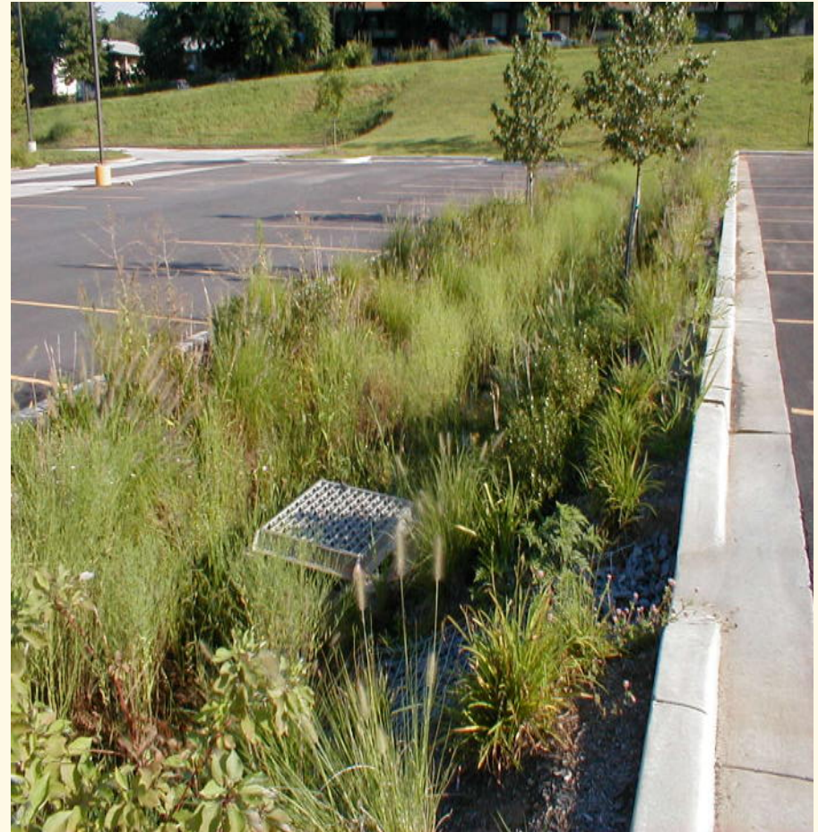
Bioswale, or recessed parking lot island designed to collect stormwater and filter it prior to release to on-site detention basin.
