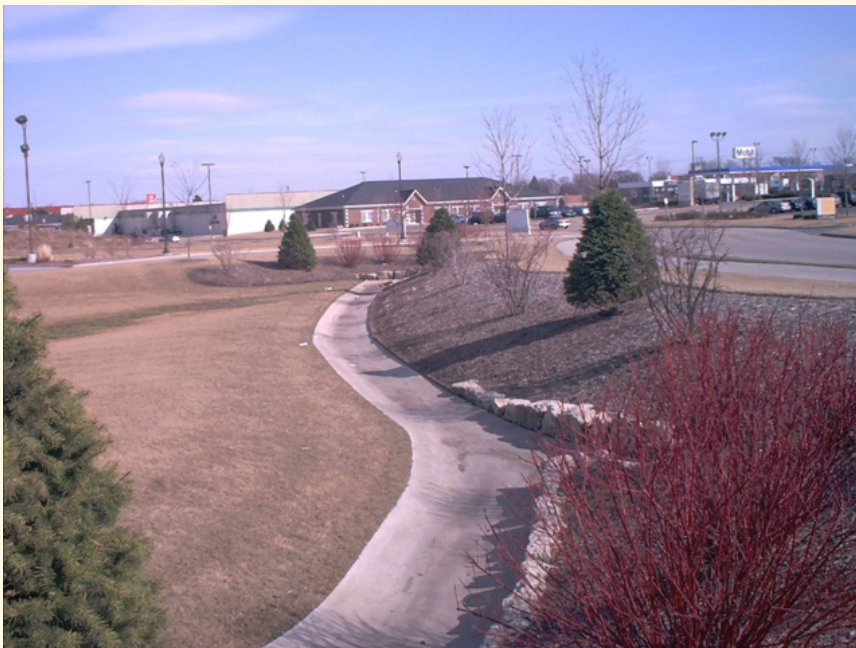
Traditional detention facility with concrete low flow channel
