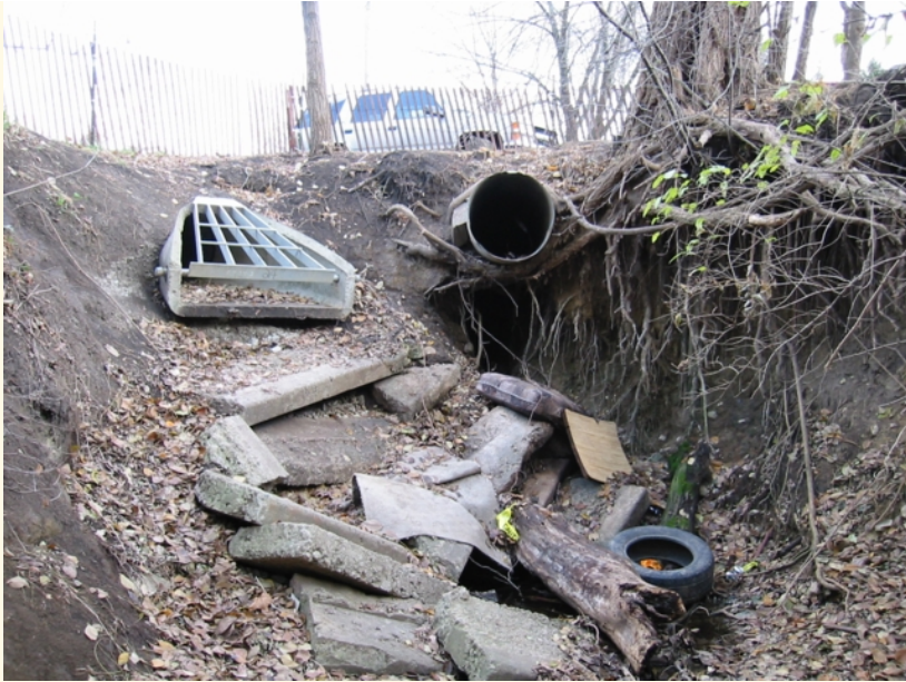
Storm sewer conveyance
