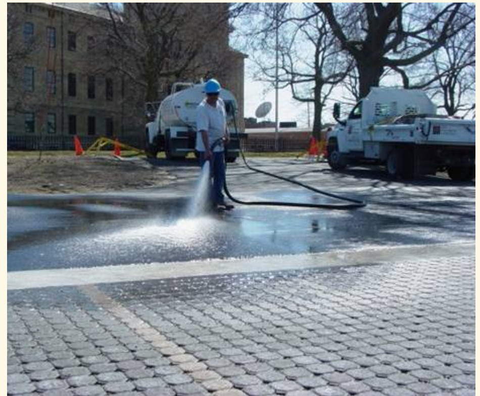
Porous pavement parking stalls adjacent to standard asphalt driving lane.
