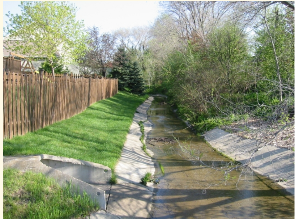
Open channel conveyance
