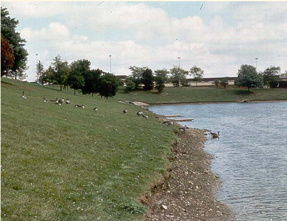
Typical detention pond ringed with turf grass. Note Canada Geese and significant shoreline erosion.
