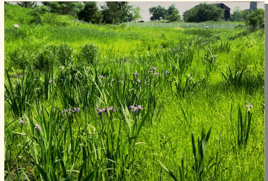
Drainage swale planted with native vegetation and designed to slow down runoff and retain as much as possible.
