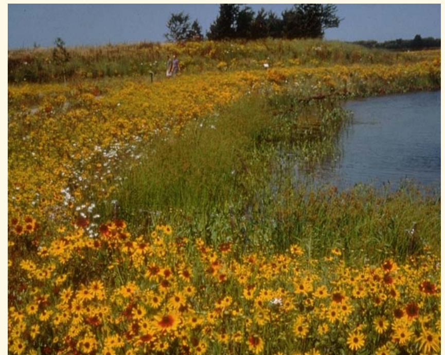
Naturalized detention with native vegetation around basin perimeter..
