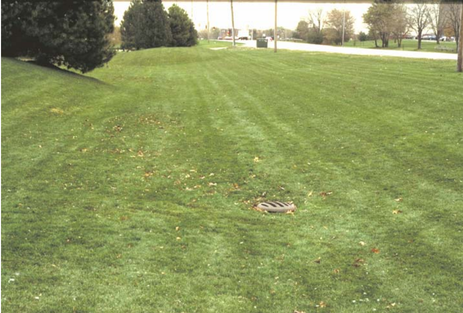
Turf grass drainage swale designed for conveyance.
