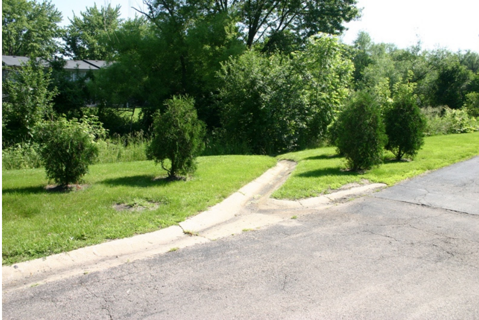
Above: Condominium parking lot runoff routed directly to Tyler Creek (Lower Tyler Creek Subwatershed).
