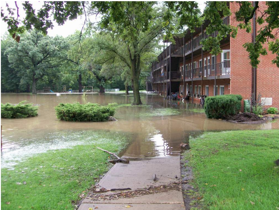
Right: Photo of flood damage to building on west side of Judson University campus following a August 2007 thunderstorm
