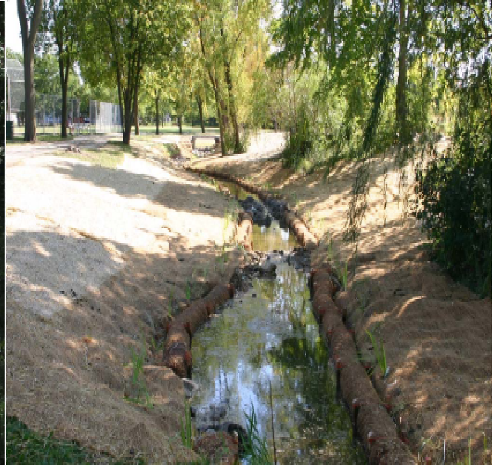
Post Construction (SW of Site)
