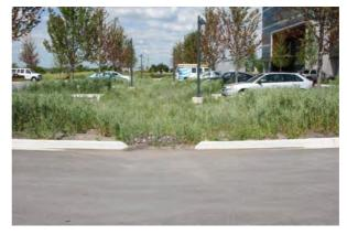
Figure 3-9. Bioretention in Office Parking Lot
