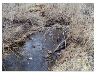
**Figure 4-17.** Side slopes of Dixie Creek Reach # 3 have subsided, and washed out streamside vegetation often accumulates in debris jams within the channel. (Source: Village of Algonquin report prepared by AES)
