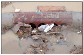
**Figure 3-23.** Accumulated sediment and debris at storm drain inlet marked "Dump No Waste; Drains to River."
