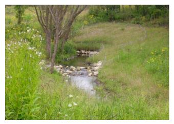
**Figure 4-25.** An example of riffle restoration which could be used to enhance and improve eroded areas along Shaw Creek. Riffle structures can increase dissolved oxygen levels, protect bank stability, and allow for balanced sediment transport through the stream corridor.
