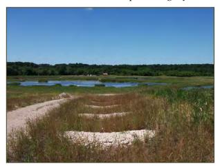
**Figure 4-8.** An example of rock checks previously installed elsewhere at the Jelke Bird Sanctuary along with a vegetated swale stabilized by native plantings. This approach could be used to stabilize eroding gullies and hillslopes in other portions of the project site.
