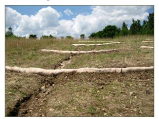
**Figure 4-7.** Although wattles were installed along a steep slope area, undercutting has continued to occur. It is recommended that rock checks be installed along existing gullies. In addition, a small berm could be constructed upstream of the gullies to store runoff and provide a potential mesic prairie / wetland restoration area. This would reduce runoff discharged to downstream areas and reduce potential gully erosion.
