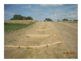
**Figure 3-2.** Soil Erosion and Sediment Control Practice: Rock and Straw Wattle Check Dams
