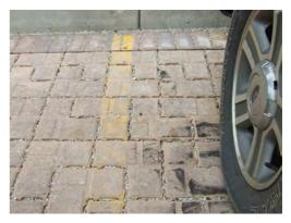
Figure 3-5. Permeable Pavers
