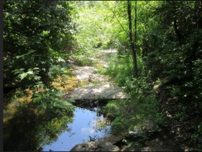
Photo 10: Concrete channel, further downstream
