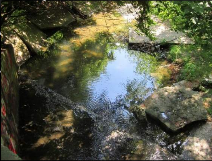
Photo 9: West of Sacramento Drive, east end of the concrete channel
