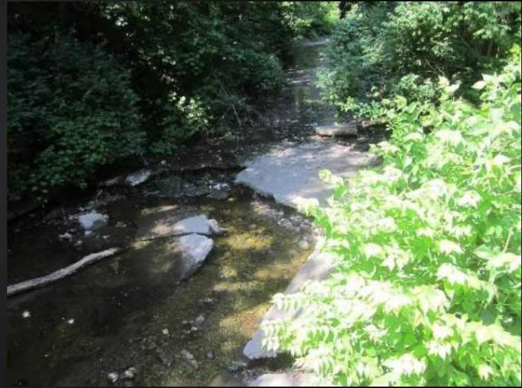
Photo 14: Western end of concrete channel looking east
