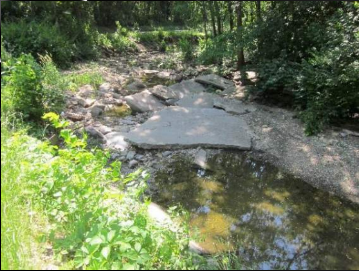
Photo 13: Near the western end of the concrete channel, looking west
