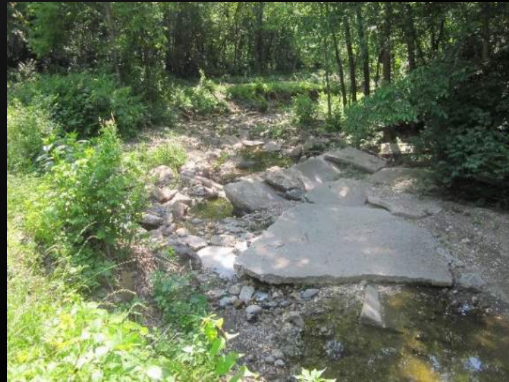
Photo 16: Western end of concrete channel, looking west, similar to Photo 13
