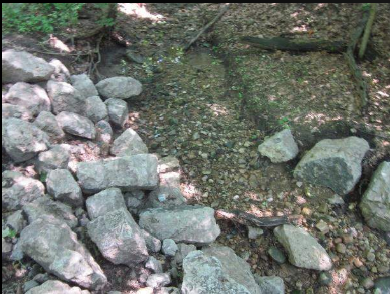
Photo 19: Side channel rip rap bank stabilization
