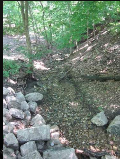
Photo 20: Side channel rip rap bank stabilization, looking NE
